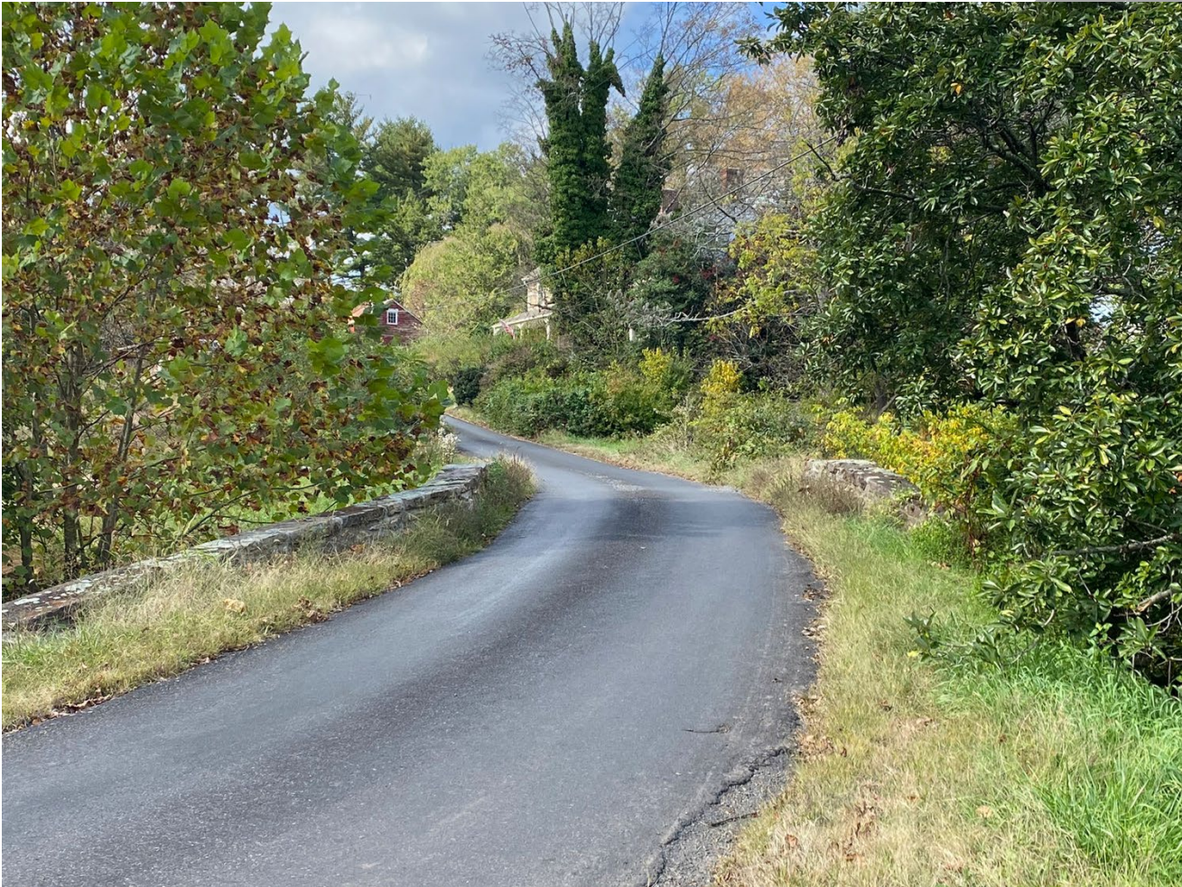
Photo 1: Yard Road Bridge, view facing northwest.
