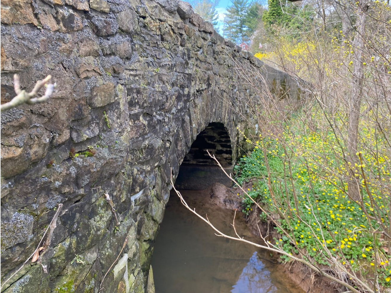
Photo 3: North (upstream) side of the bridge, view facing southwest.
