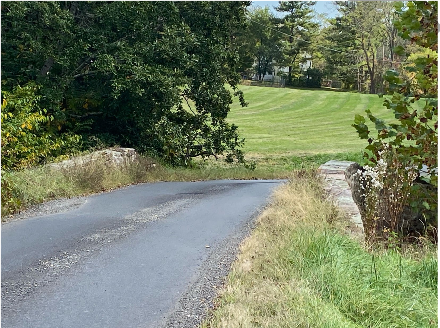
Photo 2: Yard Road bridge, view facing southeast.
