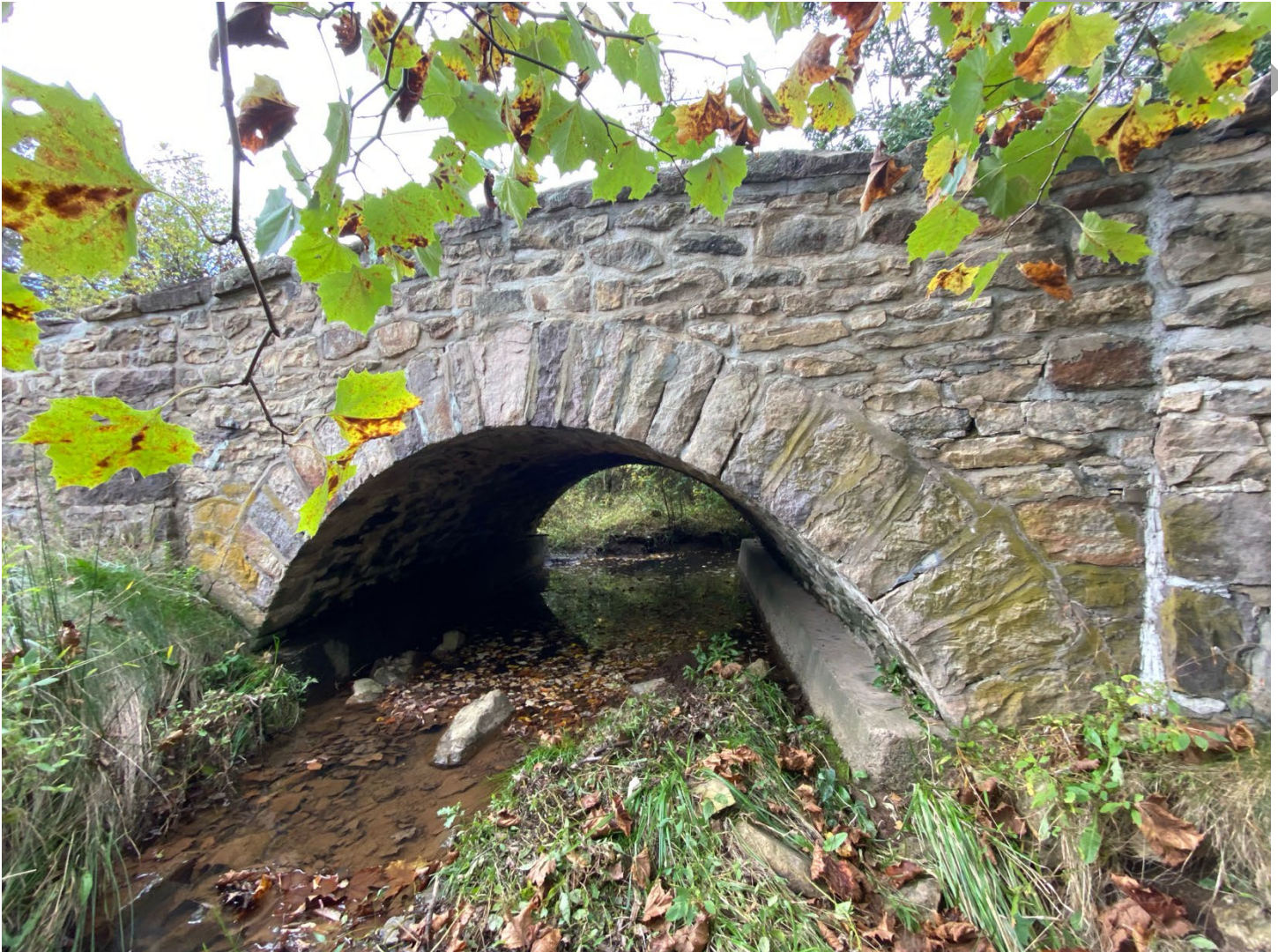
Photo 7: South (downstream) side of the bridge, view facing north.
