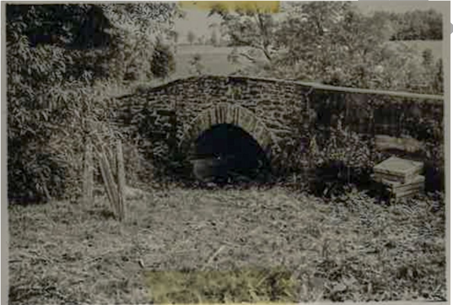
Illustration 8: circa 1940 view of the upstream side of the Yard Road bridge after the construction of the poured concrete wingwall. 8
